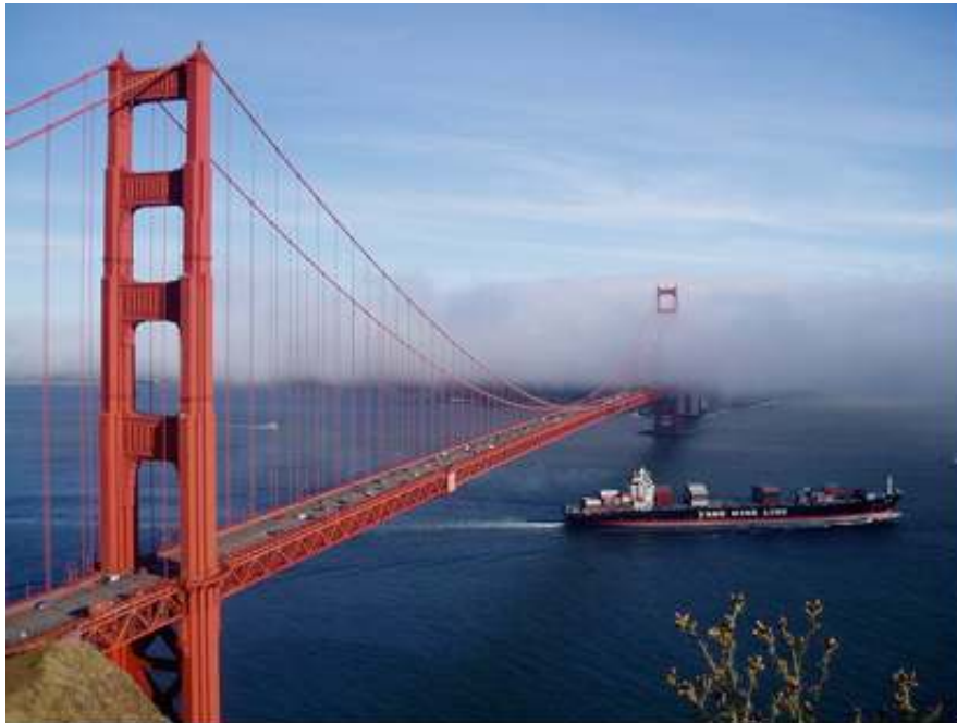
Golden Gate Bridge 1
